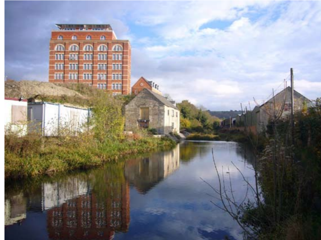
The underutilised asset of the canal, with the Hill Paul building restored and converted to flats.
