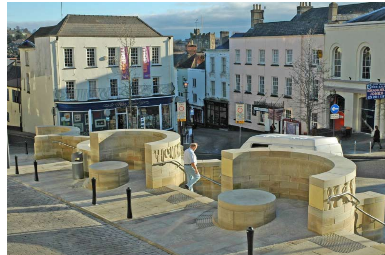
High quality public realm improvements have helped to improve the economic performance of Chepstow High Street.
