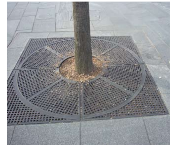
Level tree grilles bound with gravel.
