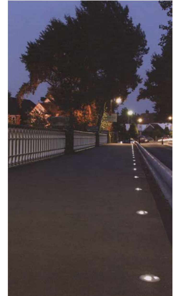
Feature ground lights can enhance key pedestrian routes at night without obstructive lighting columns.
