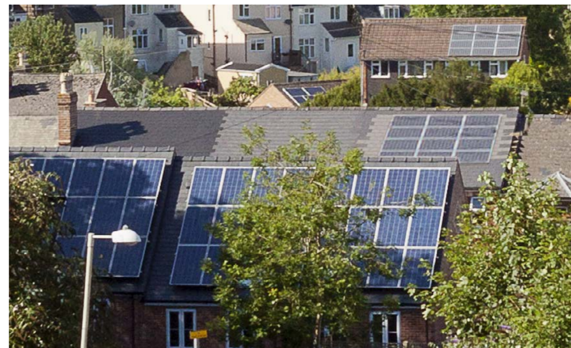
Domestic photovoltaic panels in Stroud.
