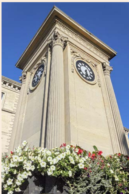
'Four Clocks' near the Subscription Rooms.
