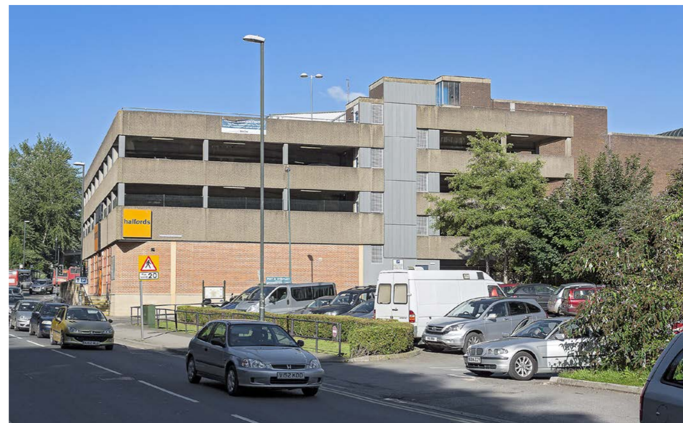
Street level and multi-storey car parks in Merrywalks.
