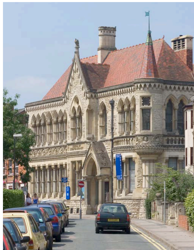
The Victorian Centre for Science and Art in Lansdown, part of Stroud's 'built and historic environment'.
