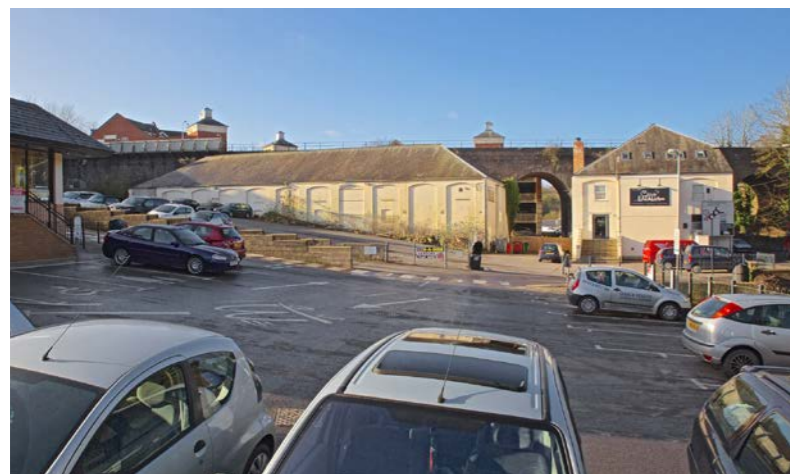
Railway arches development site.
