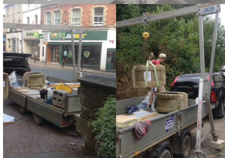
Stonemason Jonny Anderson working on the gates at Bank Gardens
