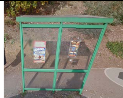
Stratford Road, opposite no. 61
